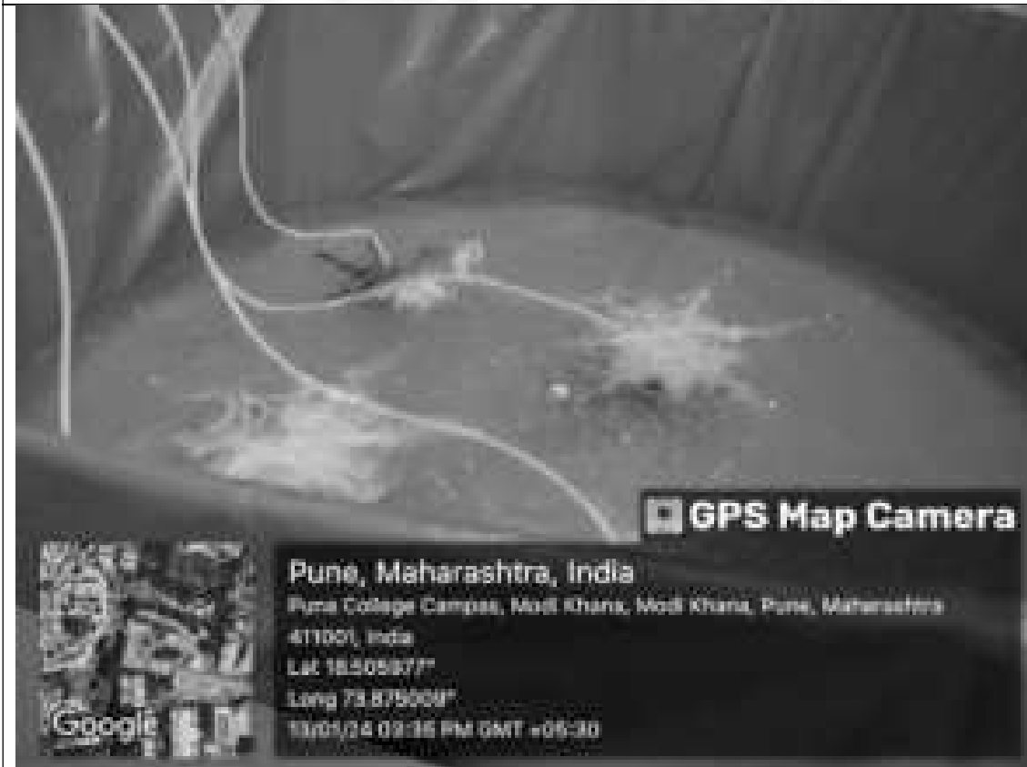
First sight of operational air blower in side the tank
