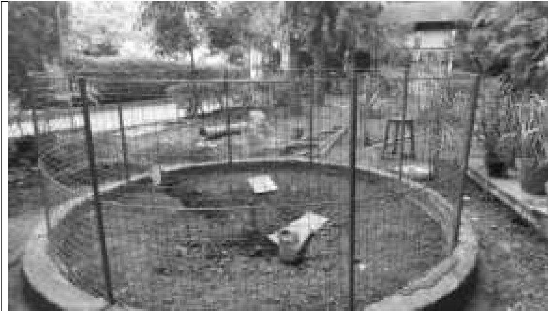
Biofloc tank: Under Construction
