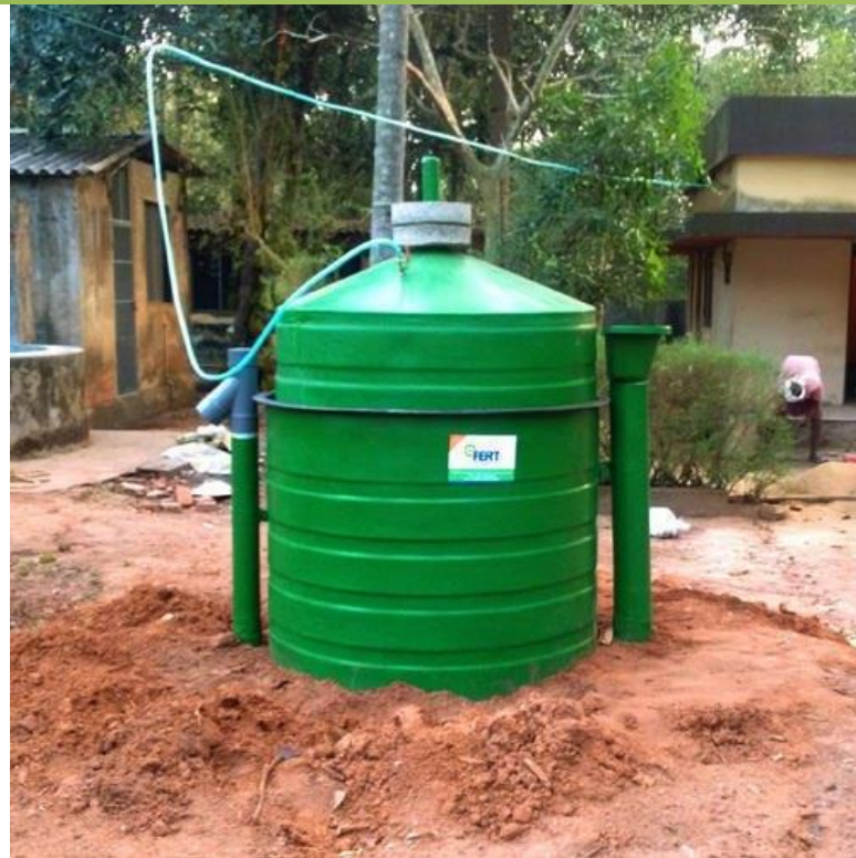
Bio-Gas Generation Plant - 10g/day- At canteen
