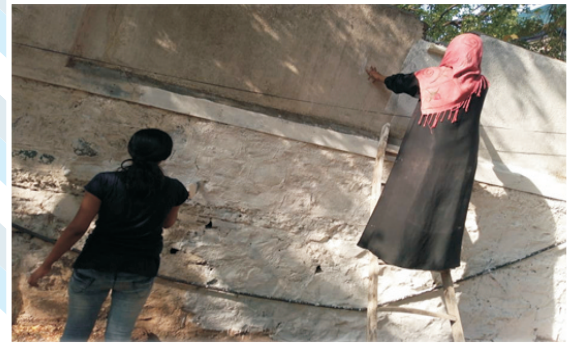
Team painting the walls
