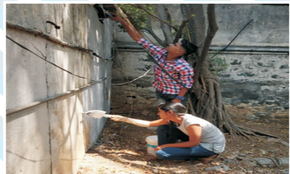
Team painting the walls
