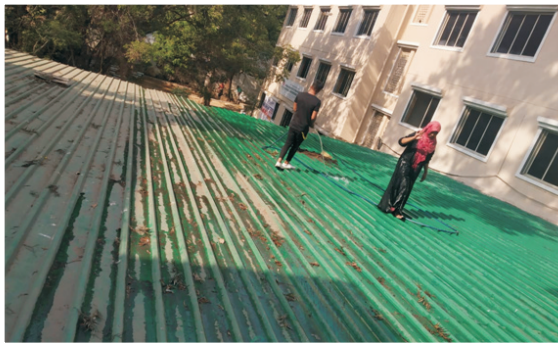
NSS Volunteers cleaning up the Ladies Common Room Roof
